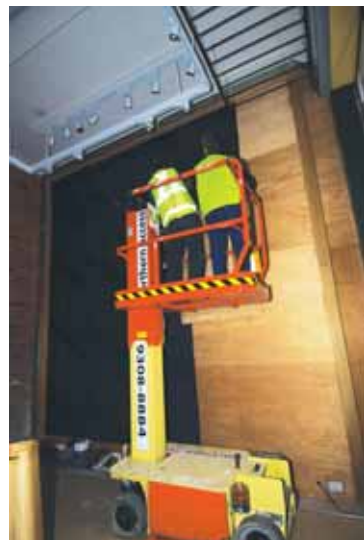
Moisture proofing the wall Self-adhesive water proofing is attached the wall to prevent moisture from penetrating the building
